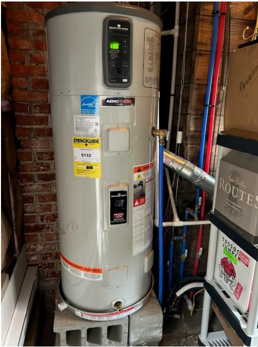
Example of Installed Heat Pump Unit in Customer’s Permanent Location
