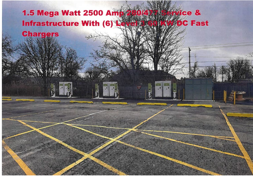
Level 3 60KW DC Fast Chargers With V2G & Management Program with will allow you to charge at any time or charge Rate.
